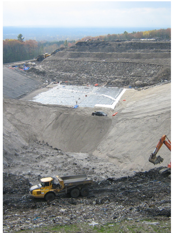
Figure 4 – Tight working area and steep slopes, waste fill in background, new cell in centre, waste excavation in foreground (2009).
