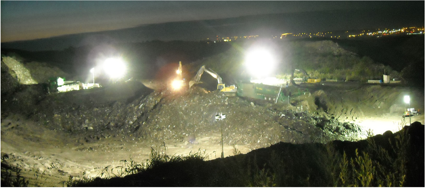
Figure 7 – Waste excavation and direct haul operations undertaken at night to limit odour impacts (2010).
