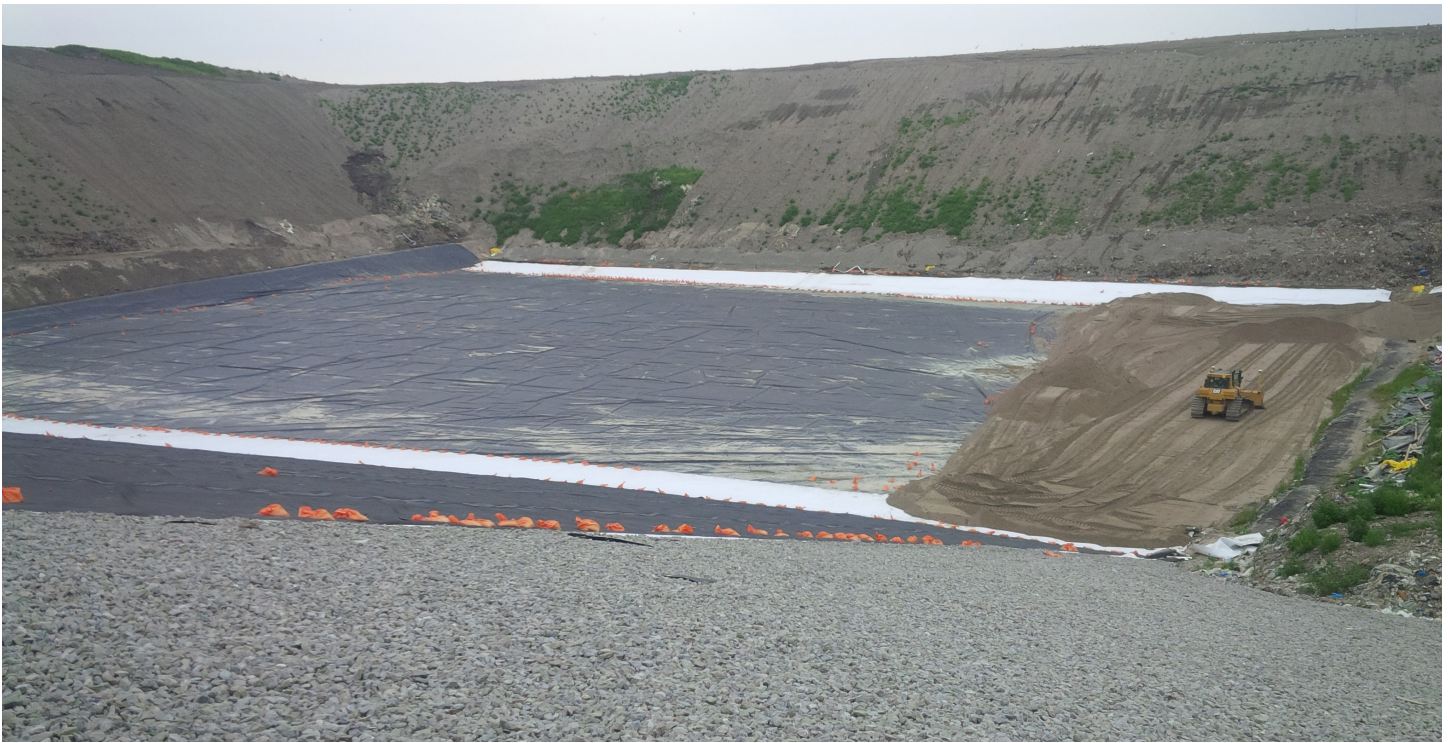
Figure 3 – Construction of the final phase of geosynthetic liner (2015).
