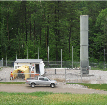
Figure 5– Landfill gas flare and plant..
