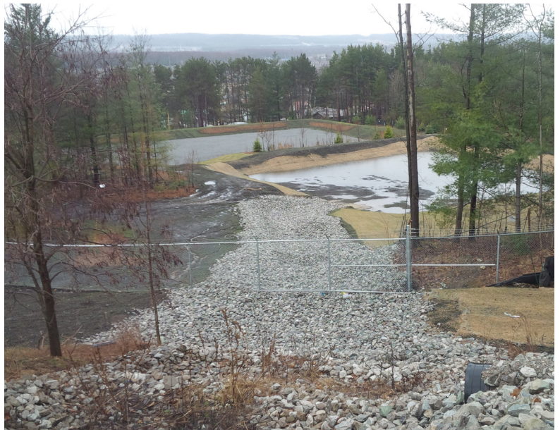
Figure 8 – Stormwater ponds control runoff and promote groundwater recharge (2016).
